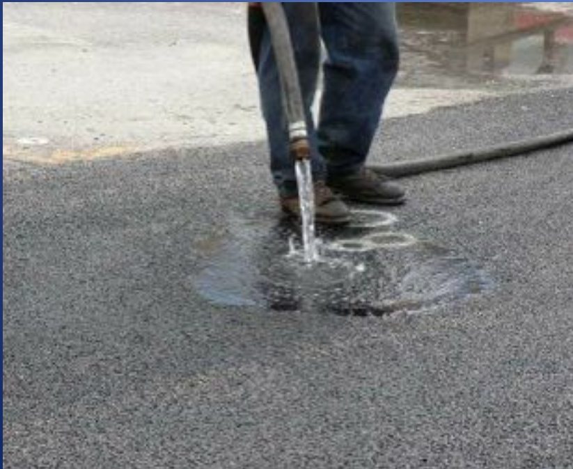
Porous Asphalt
