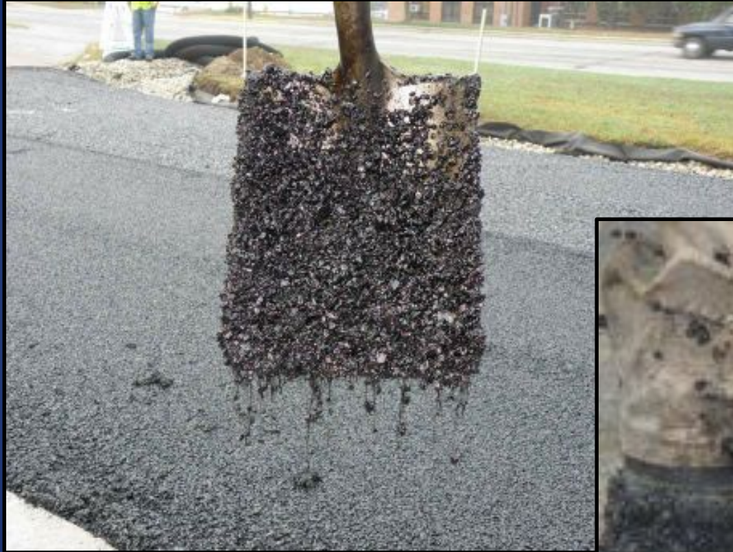
Beach Road Porous Asphalt
