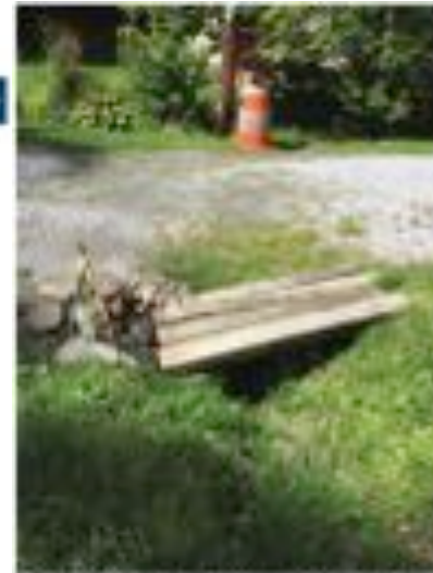
Block and culvert used to divert runoff to nearby brook on Talmadge Trail North. Photo is courtesy of Tetra Tech, Inc.
