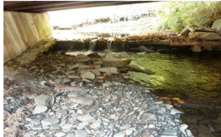
Eroded conditions at Bonnie View Avenue Bridge
