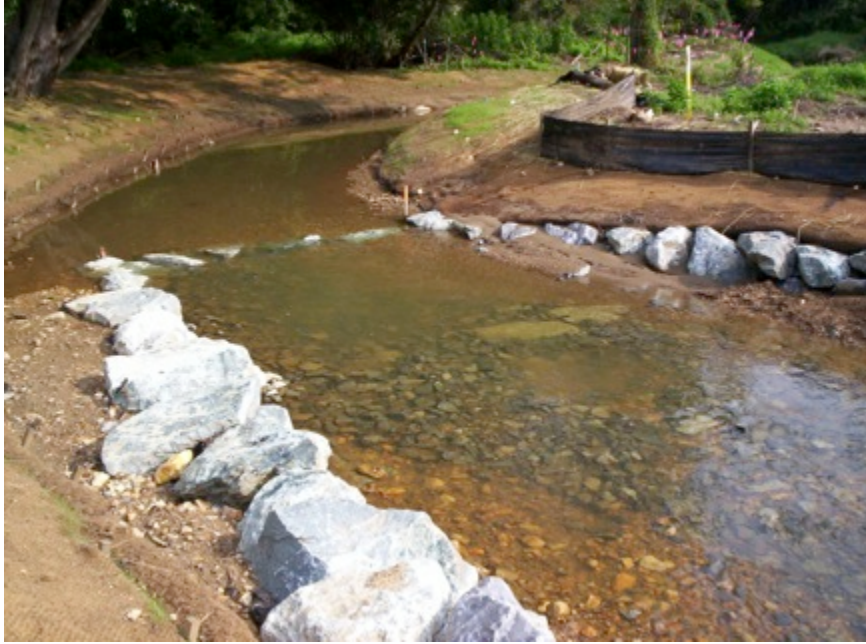
Newly Installed Cross Vane
